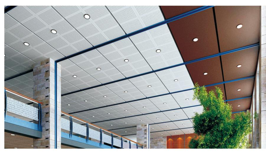
Perforations are commonly seen on metal ceilings, reducing noise and creating a comfortable space. To stick acoustic paper or mineral wool to the back of perforated ceilings is very conducive to add absorbed dose of an enclosed space, and further reduce noise pollution. Below are different types of perforations. Each type can be done in various open area ratios to fulfill different acoustics. Additional perforations and sizes are available as custom options.
